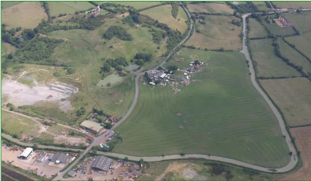
Part of former Napton Brickworks site (to the left in the photo) with Oxford Canal in the foreground
